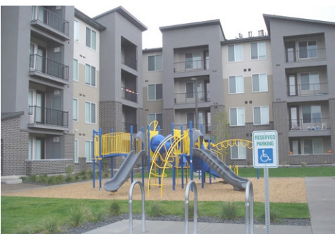
Figure 2.19 - Affordable housing development example, Enclave at 1400 (jobs.utah.gov)
