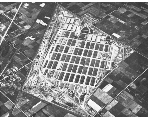
Figure 3.17 - From its initial construction, local traffic has been routed around the Freeport Center and adjacent industrial areas
