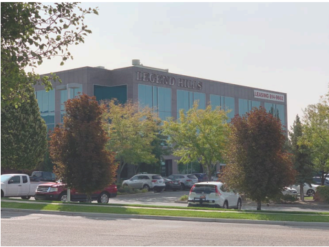
Figure 2.1 - Site of Legend Hills office park, with potential for future development. (September 2020)
