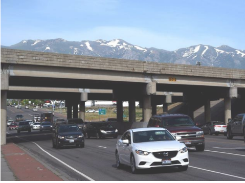
Figure 3.5- The I-15 overpass at the 700 South/State Route 193 interchange
