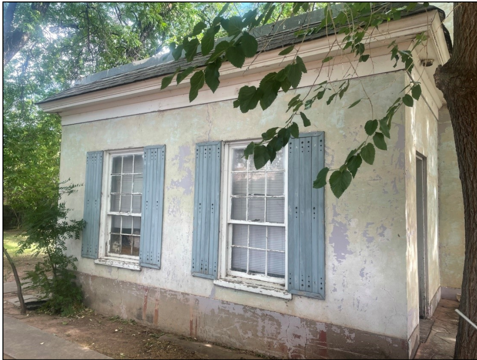
In-period addition on north elevation; looking southeast
