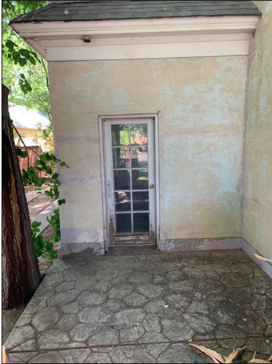
In-period addition on north elevation; looking east
