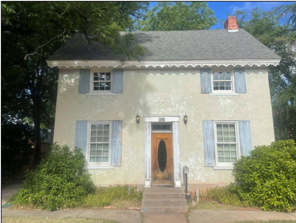
Primary façade (west elevation); looking east
