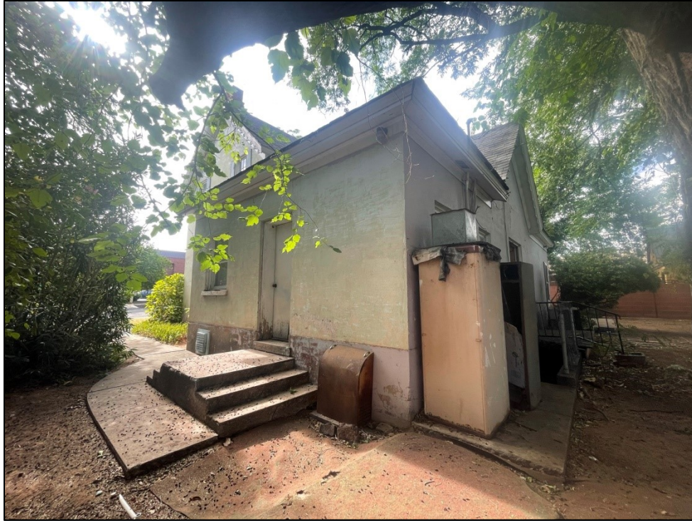
South elevation (at left) and east elevation (at right) showing in-period addition; looking northwest
