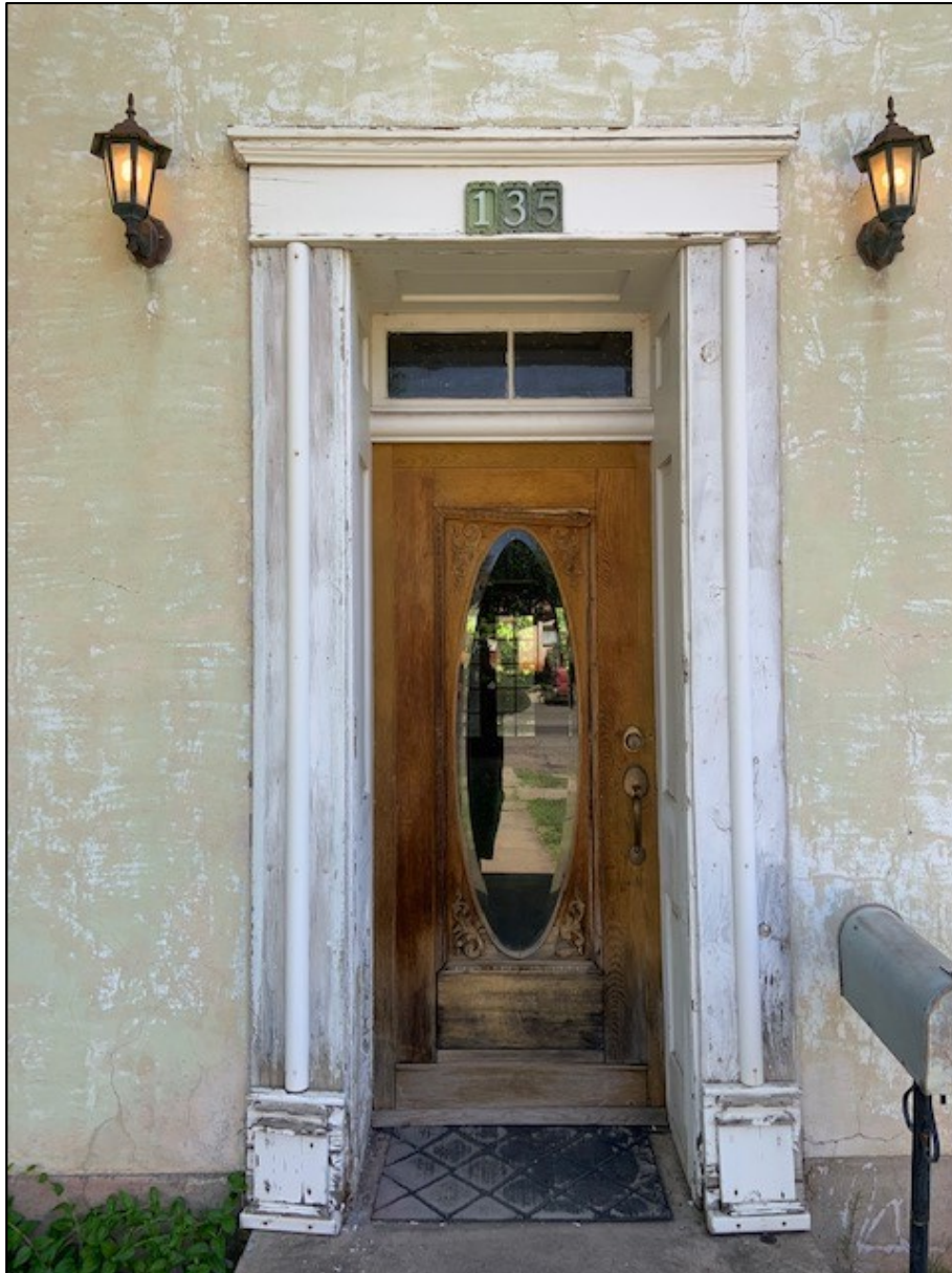
Recessed entry in primary façade showing historical detail; looking east
