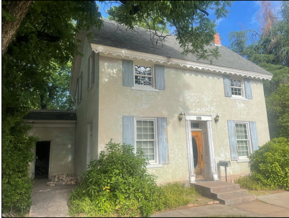
Primary façade (west elevation) at right with north elevation at left; looking southeast
