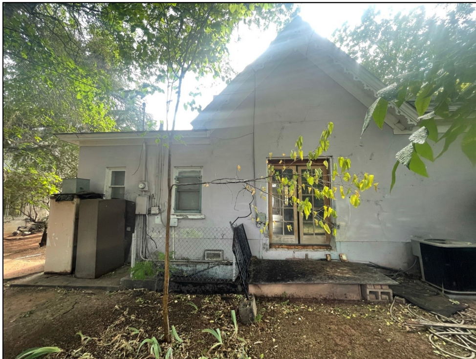
East (rear) elevation; looking west
