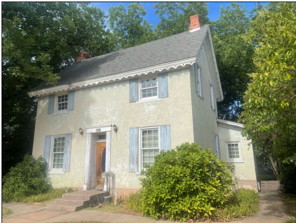
Primary façade (west elevation) at left and south elevation at right; looking east
