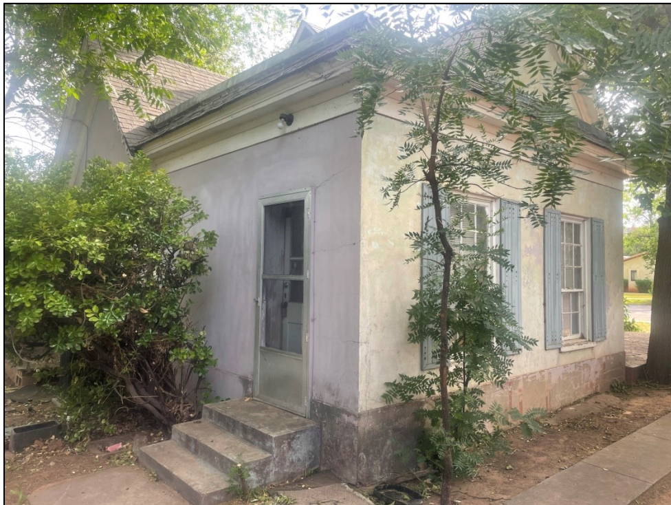
North elevation (at right) and east elevation (at left); looking southwest
