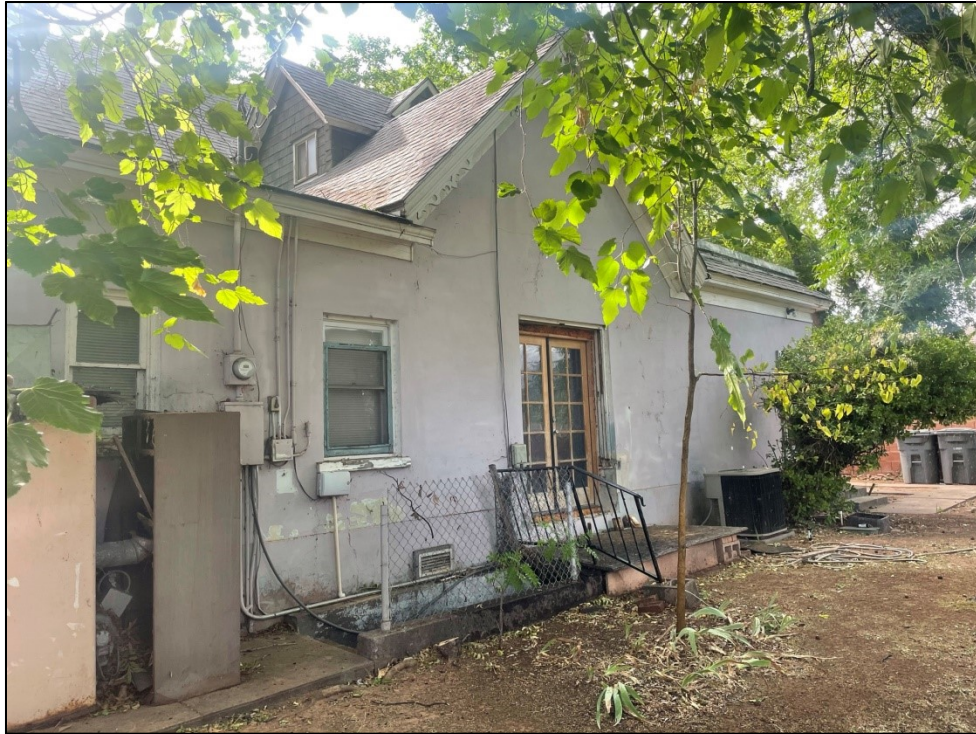
East (rear) elevation; looking northwest
