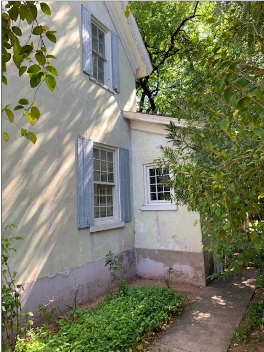
South elevation showing in-period addition; looking east
