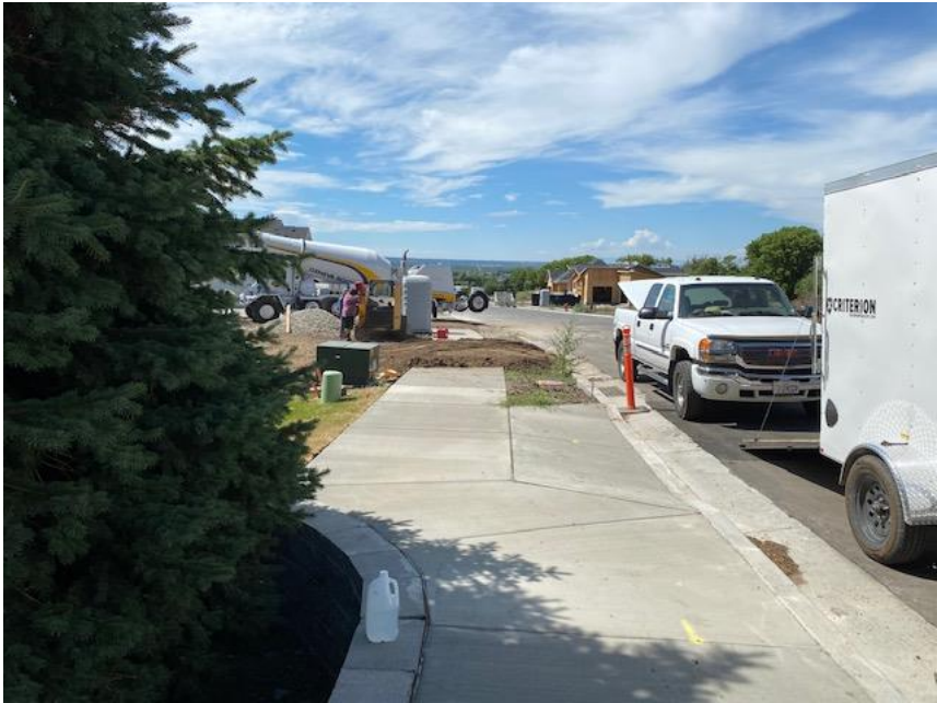
View looking south as the sidewalk moves away from the curb with a standard park strip
