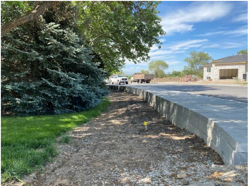
View looking south showing the height of the retaining wall at the back of curb
