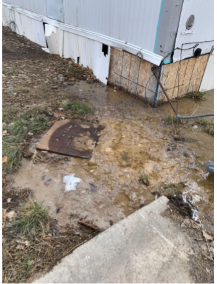
Image 3: Major sewer Leak in Melody Estates Mobile home park, Example of high density housing issue.
