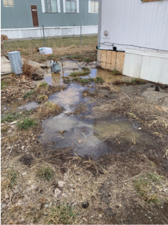
Image 3: Major sewer Leak in Melody Estates Mobile home park, Example of high density housing issue.
