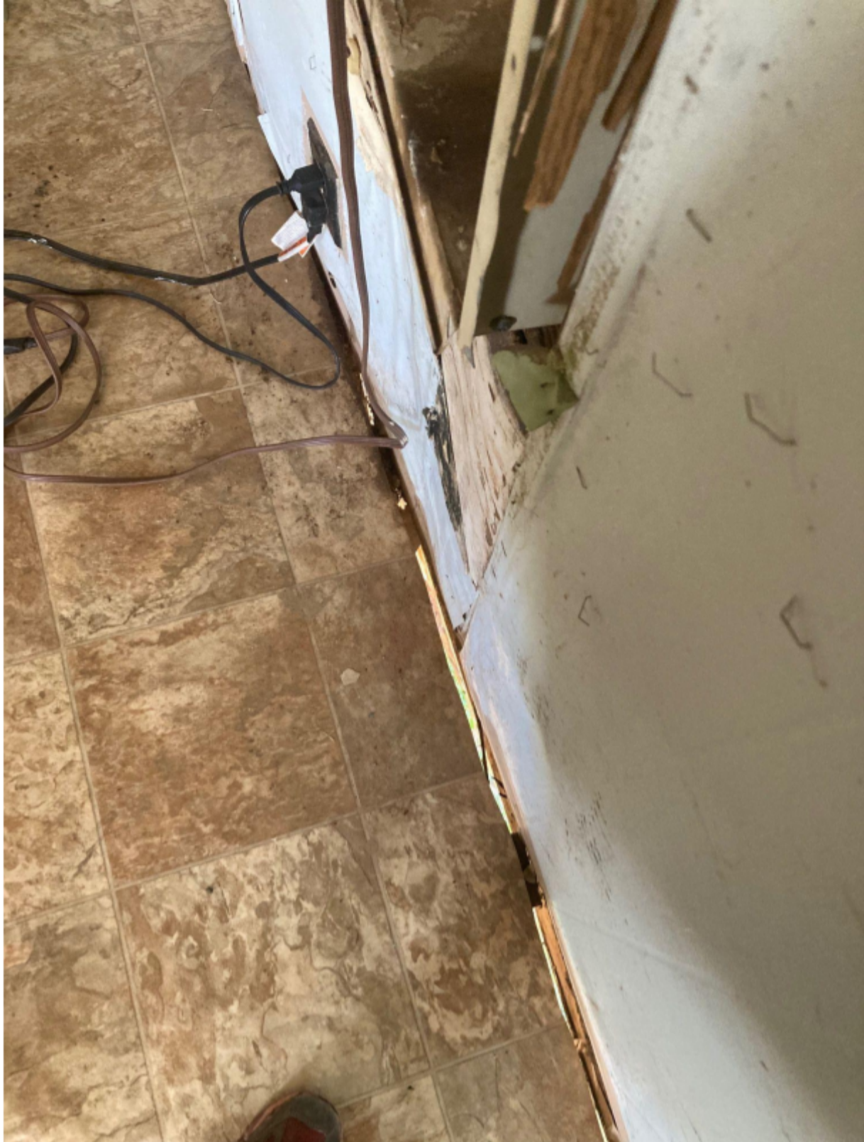
Image 1a: Walls separating from a rented trailer floor and frame in Moab.
