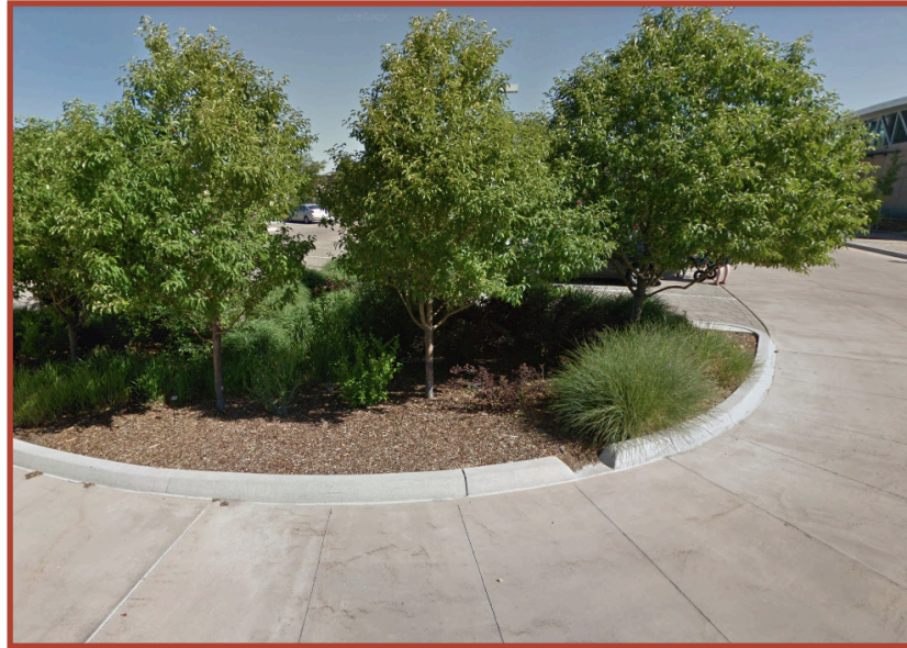
Parking Lot Curb Cut to Manage Stormwater Runoff from the Impervious Surface
