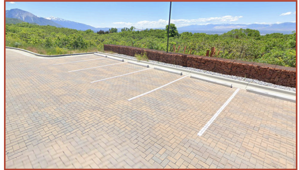
Pervious Paver Parking Lot
