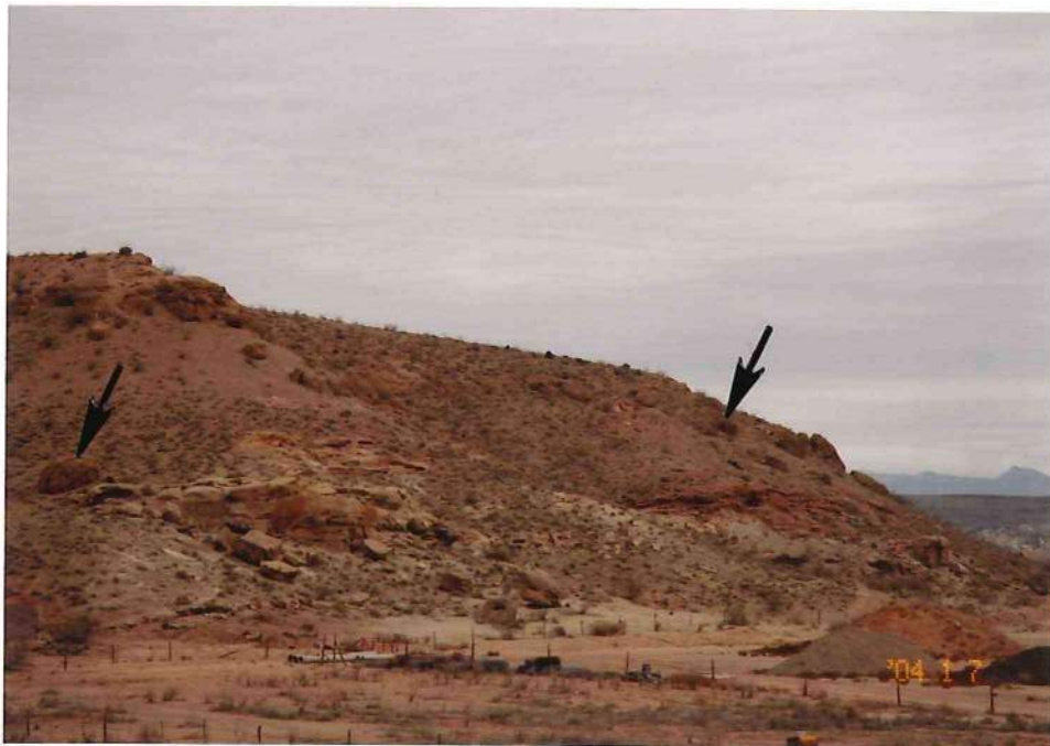
Photo Exhibit 3 - View of southern portion of the site looking northeast. Some conglomerate boulders have broken off and rolled or slid down the slope (see arrows).
