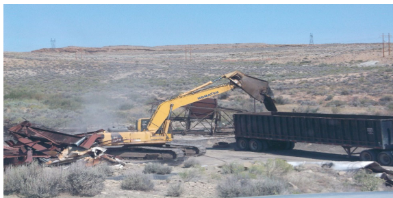
Metal & Debris Separated for Reuse or Recycling
