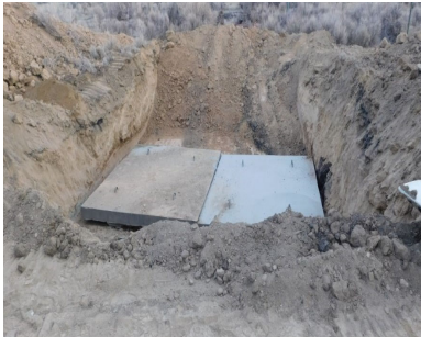
Cap Placement on Bedrock
