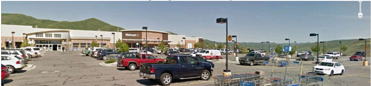
16 Foot Tall Lighting Poles, Park City Walmart
