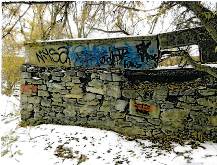
Photo 4 Missing Mortar
