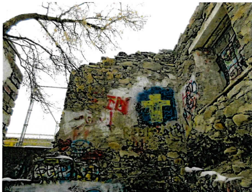
Photo 8 Unbraced wall
