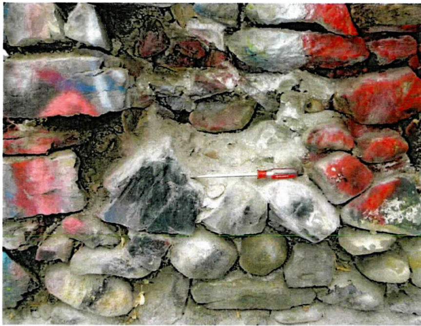
Photo 11 Deteriorated mortar
