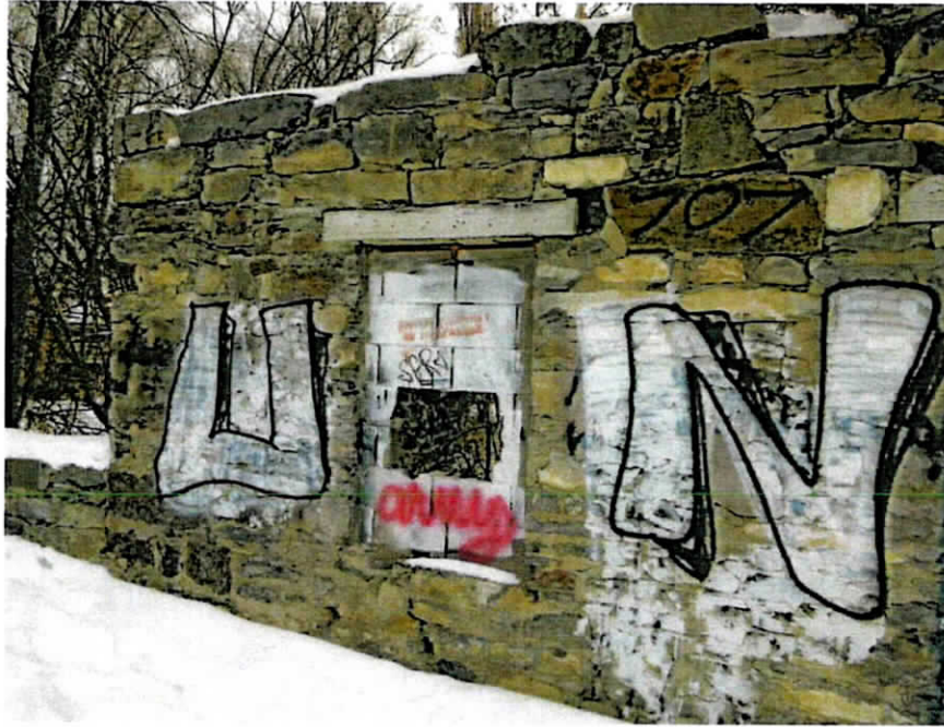
Photo 1 CMU masonry infill
