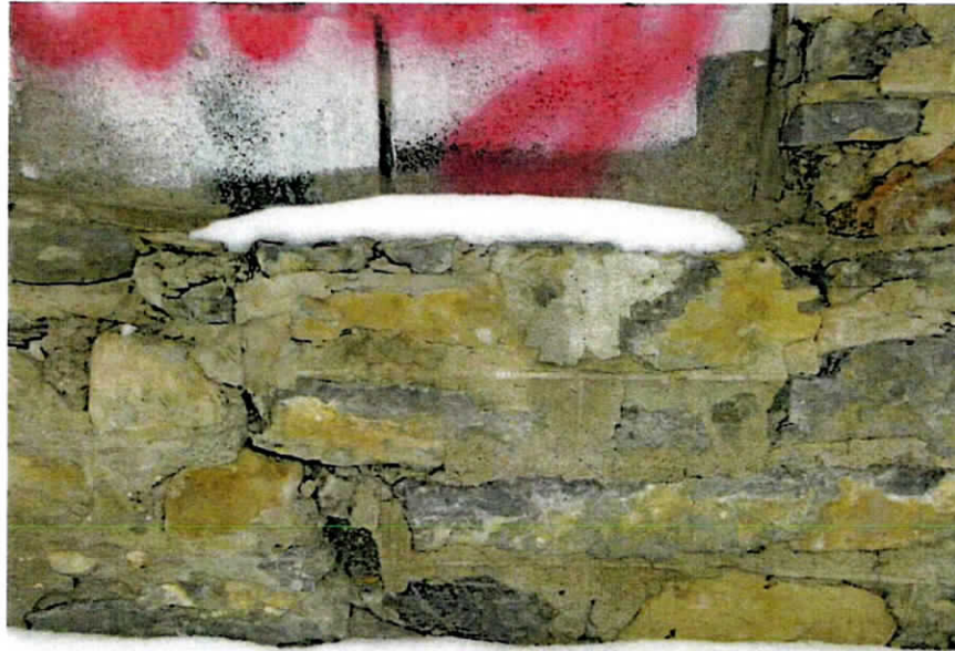
Photo 3 Missing mortar
