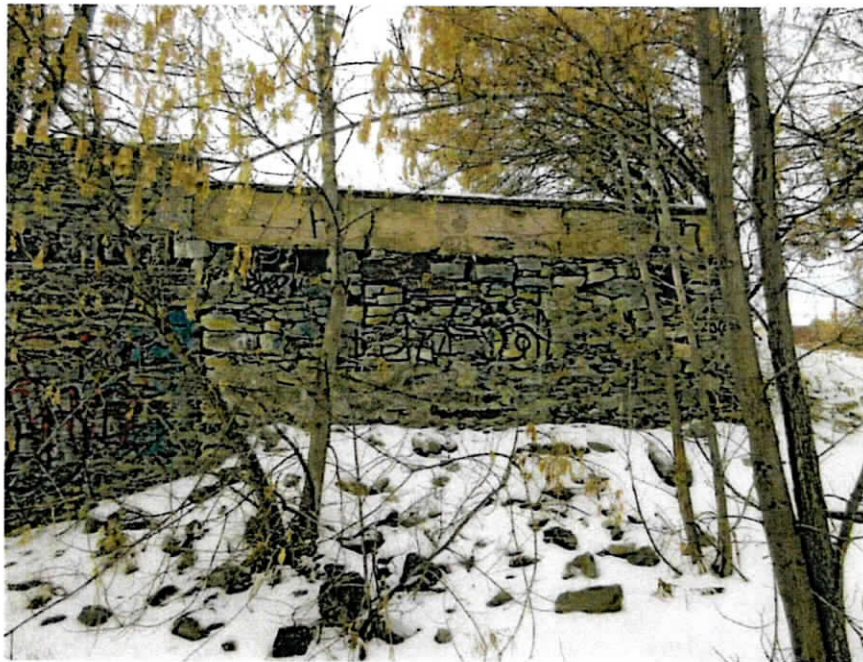
Photo 6 Missing mortar
