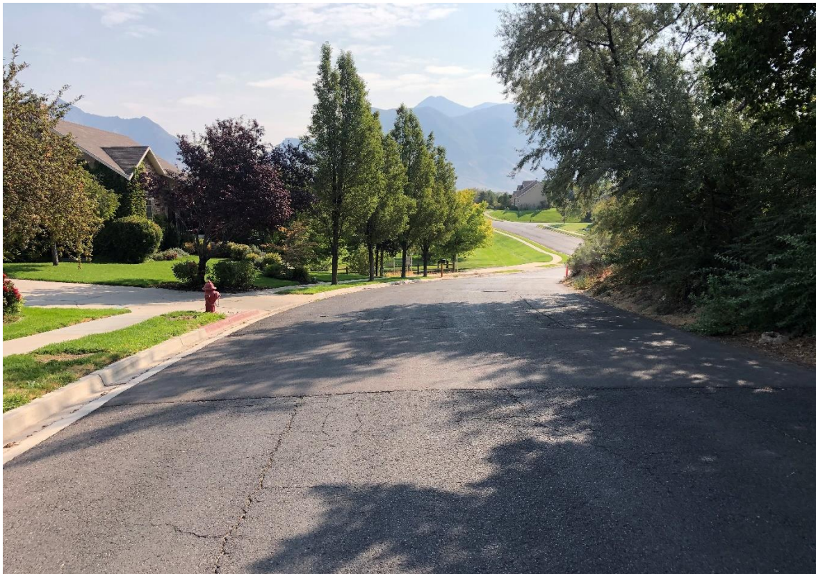
Figure 3b: Proposed Subdivision Entrance at 10250 North (Looking East).
