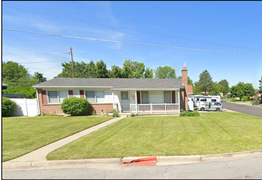
Front View (West)
