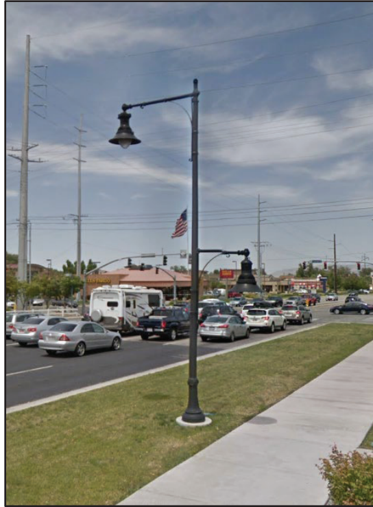
Existing streetlight to the north of proposed facility (Zions Bank)
