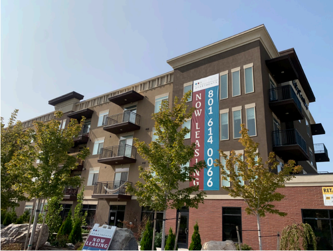
Figure 1.9 New housing constructed in Clearfield along State Street.
