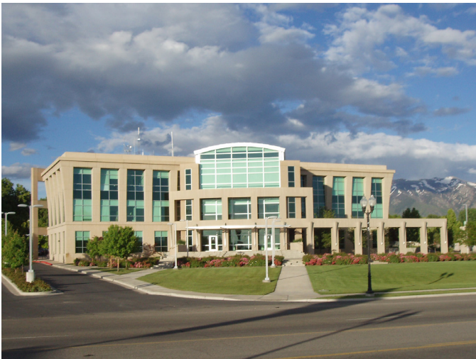
Figure 1.8 Clearfield's City Hall.
