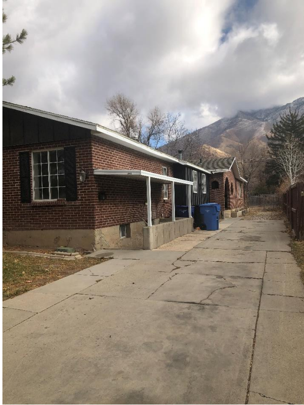
View showing basement entrance and entrance to primary dwelling
