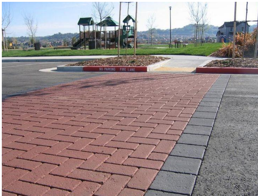
Fig. 9 stamped and colored asphalt.
