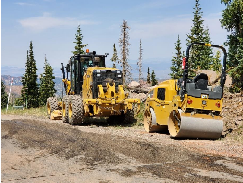
Equipment parked after applying road base on Look Out Circle
