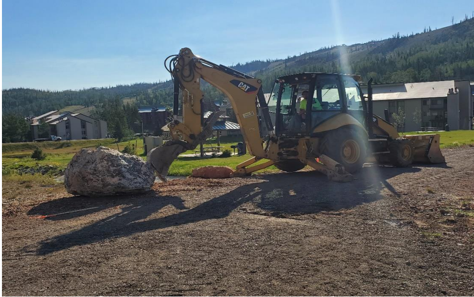
Rocks being removed as part of the Trail project around the pond
