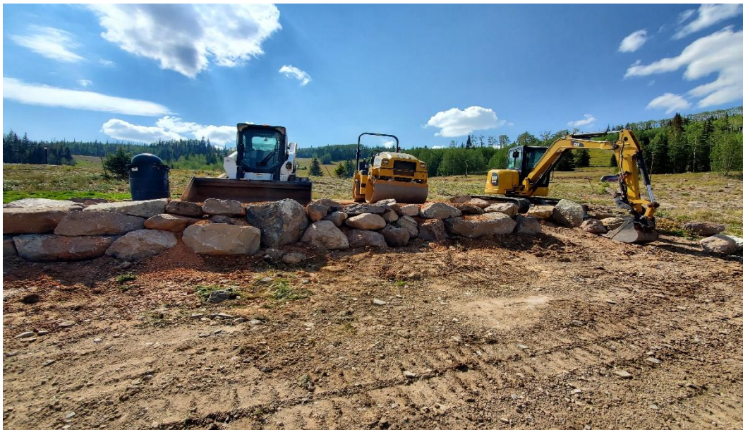
Rock wall re-redone and pad extended to fit pavilion
