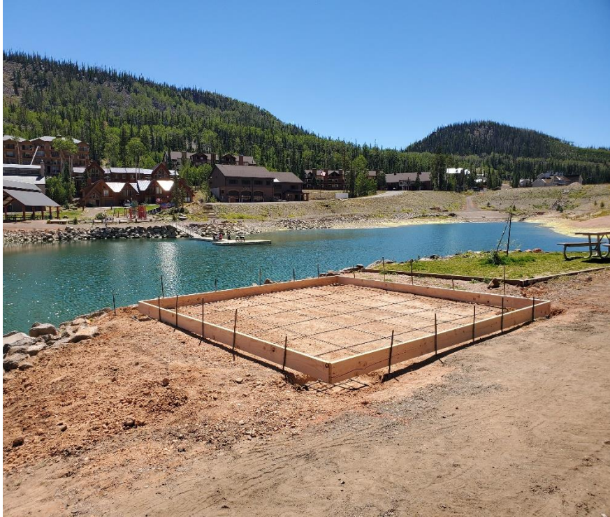
Pavilion Pad ready for cement
