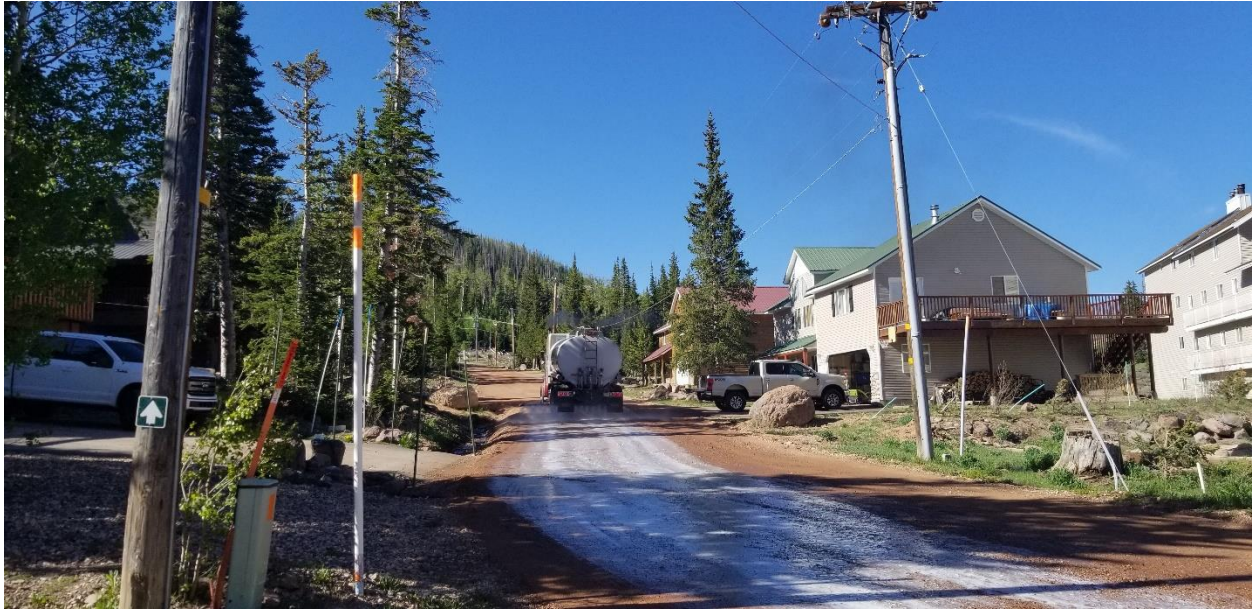
Mag Chloride being installed
