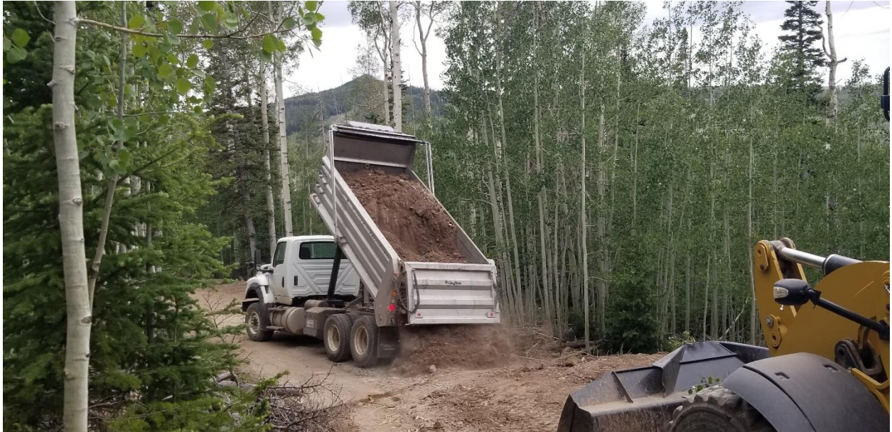
Sub grade being installed
