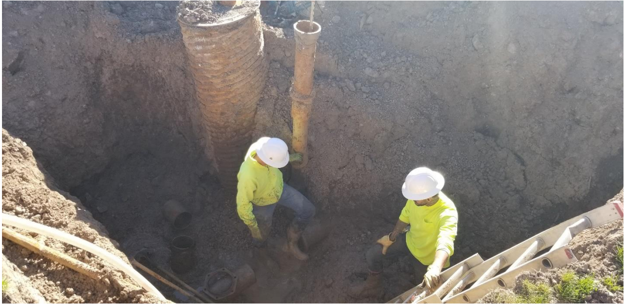
Valve install for PRV
