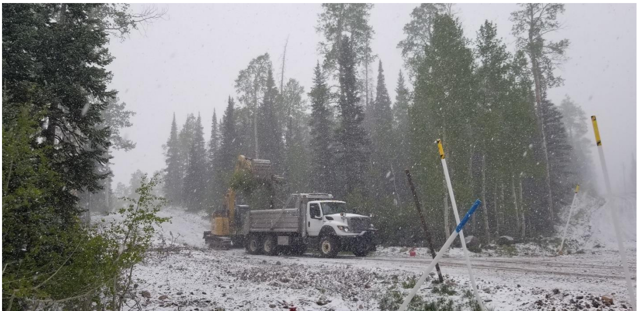
Slash removal on Street project
