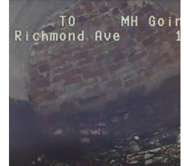
Walled-Off Pipe
