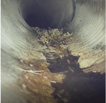
Cracked Pipe
