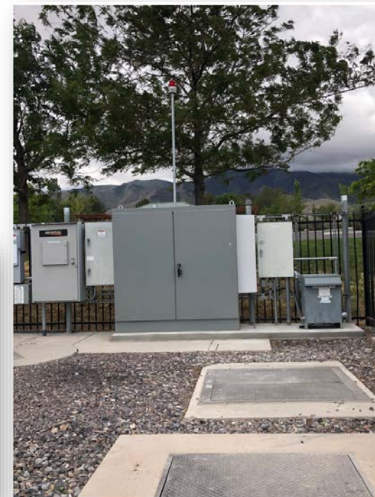
New Drive at Lift Station #6
