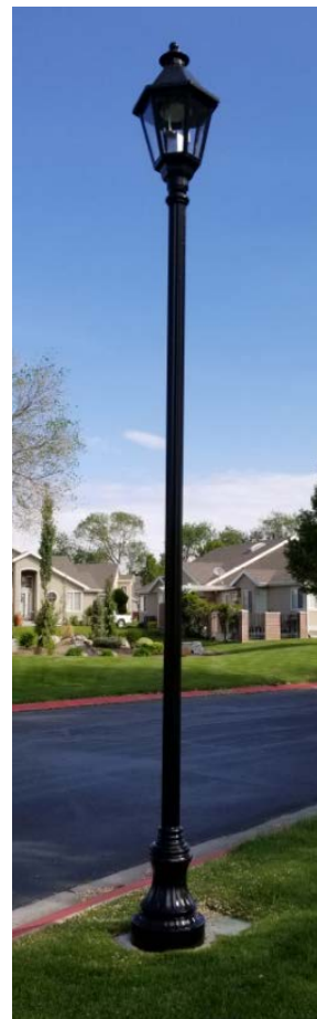
Repainted Pole in SSD
