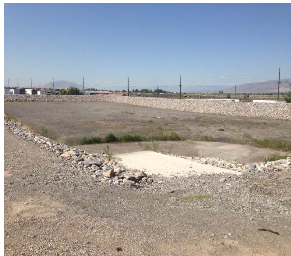
800 North Detention Pond
