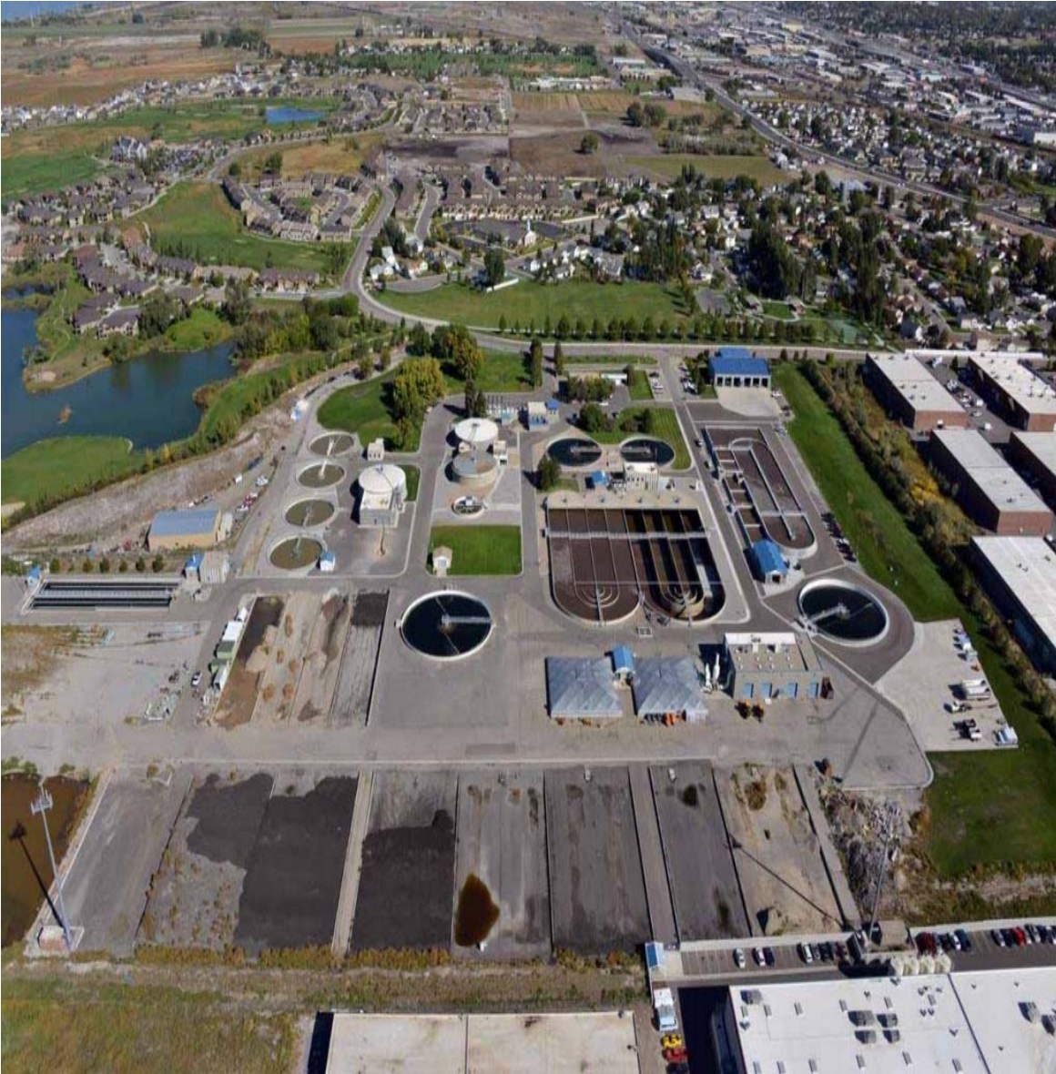
Water Reclamation Plant
