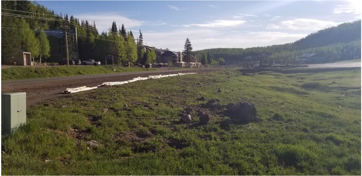
Zig Zag Fence Install
