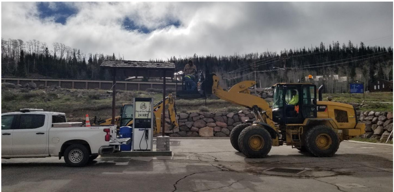
Repair Work from Wind Storm
