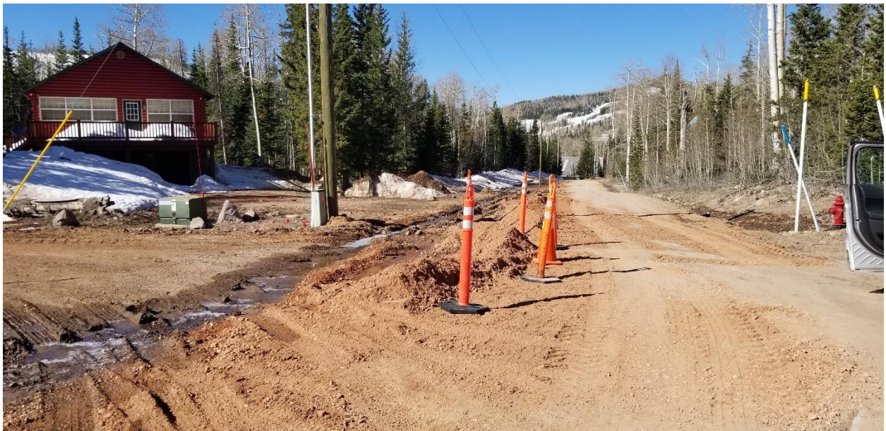
Road Work Mountain View
