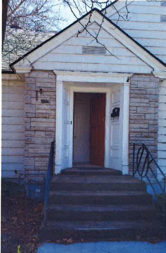
Existing Front Entry
