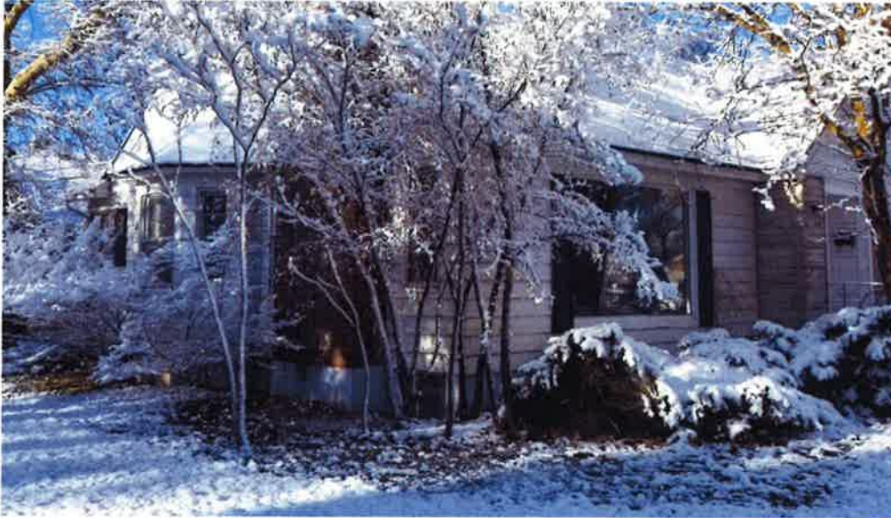
Overgrown and nuisance trees and shrubs
