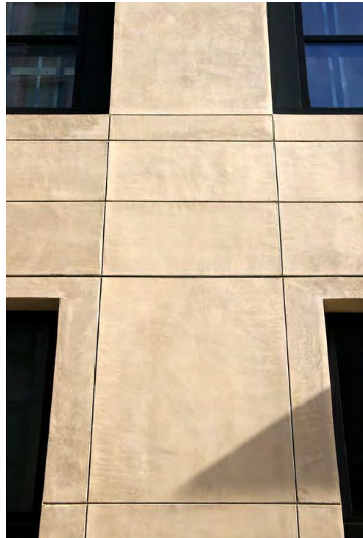
5 BASE/GABLE MATERIAL- CEMENT PLASTER SCALE: NTS
