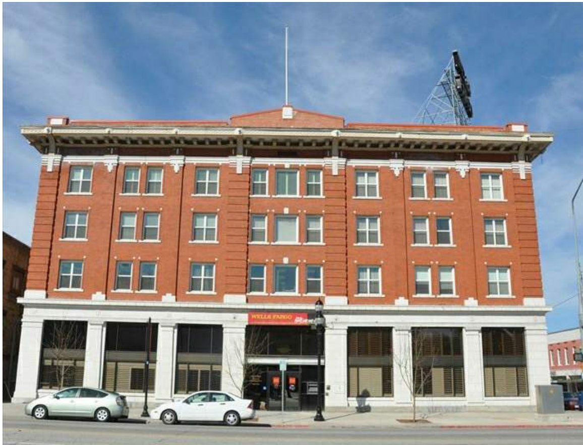
FORMER WELLS FARGO BUILDING
