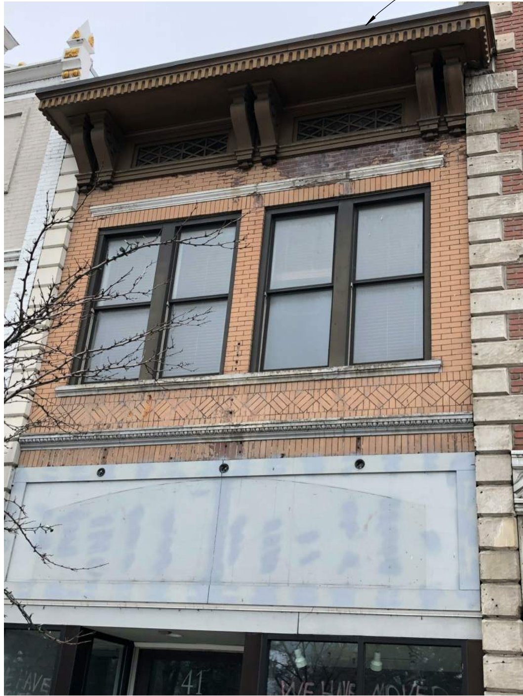
EXISTING BUILDING TO BE REMOVED
