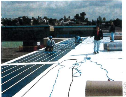
Figure 2: Cool Roofs with Solar Panels in San Diego
