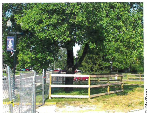
Figure 4: Fences Protect a Tree During Construction
