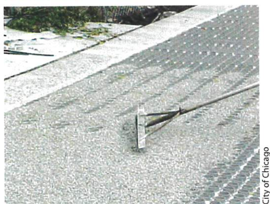
Raking gravel into a Gravelpave2 system.
