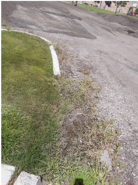
Figure 14. South Parking Lot Curb and Gutter
