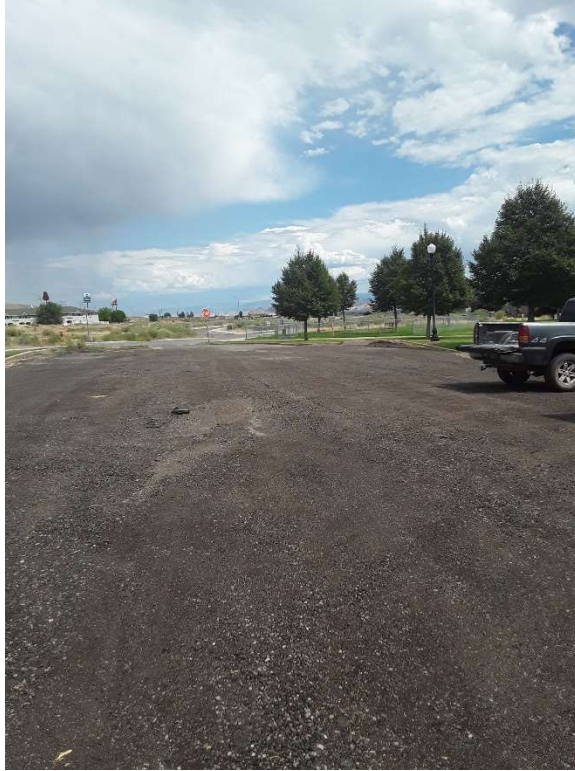
Figure 8. North Parking Lot
