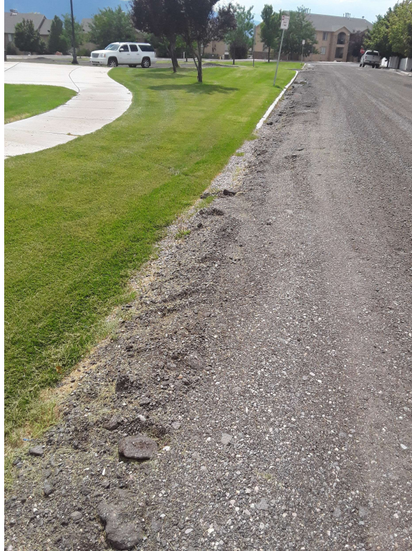
Figure 15. Centennial Park Drive Curb and Gutter
