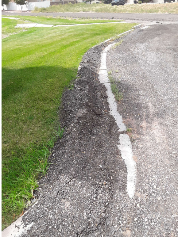
Figure 13. North Parking Lot Curb and Gutter
