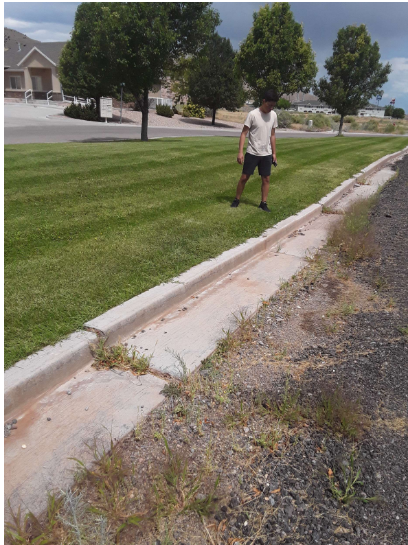
Figure 12. North Parking Lot Curb and Gutter
