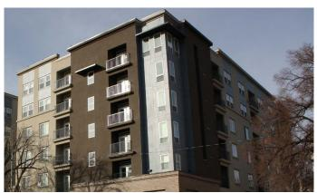
Figure 6.13 (3). Balconies Integral to Facade.
