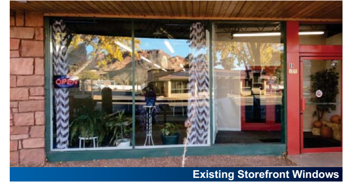
Existing Storefront Windows
