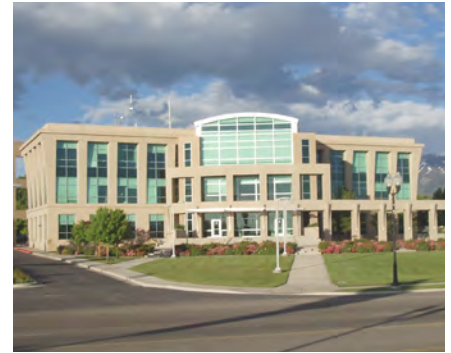
Clearfield City Hall.
