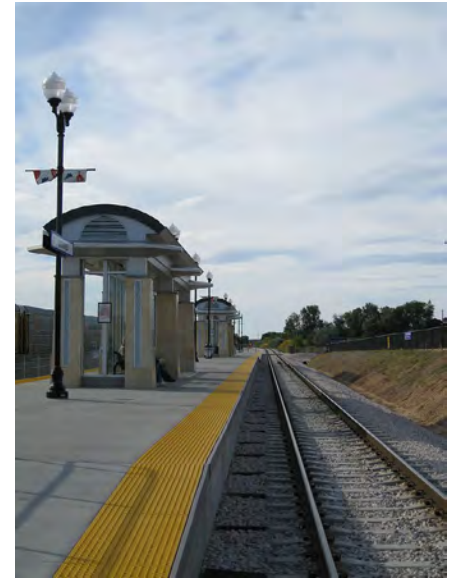
Clearfield FrontRunner Station. Clearfield City.
