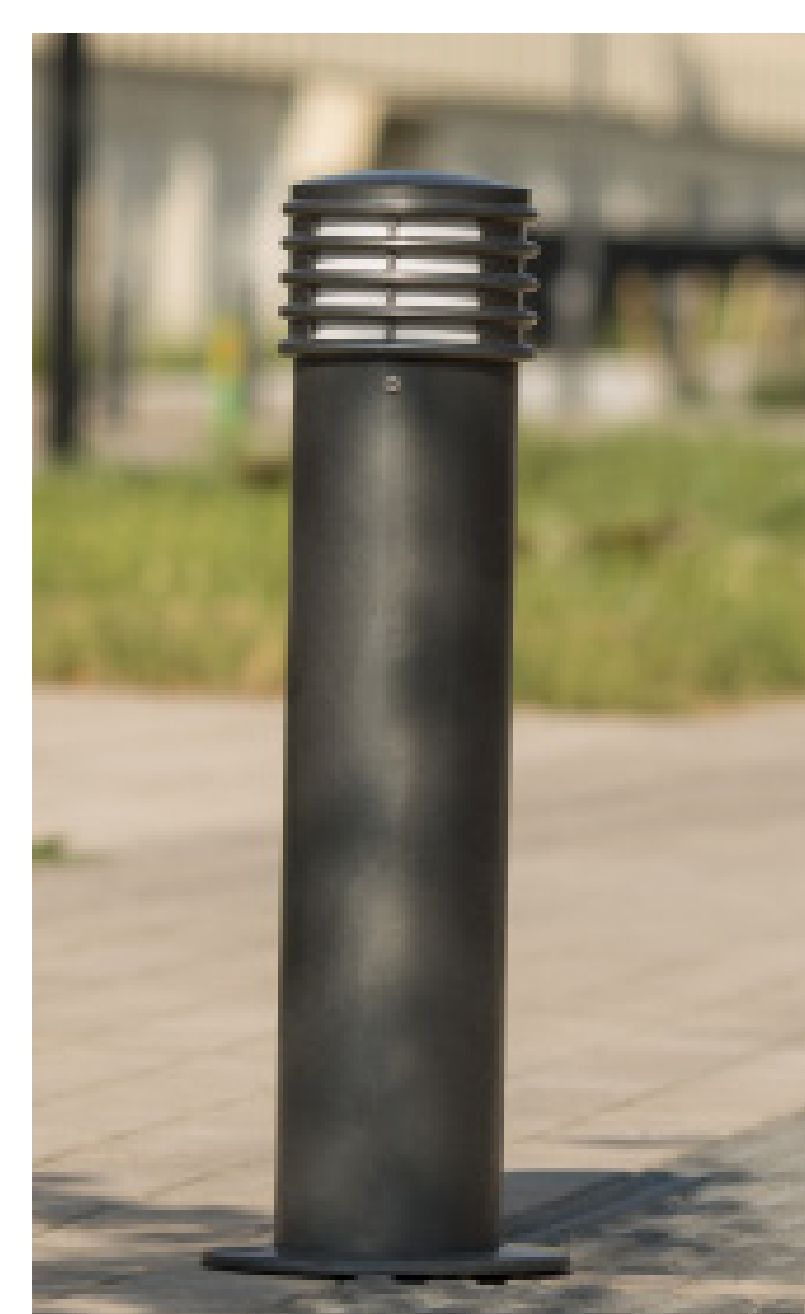
13 lighted bollard along path
