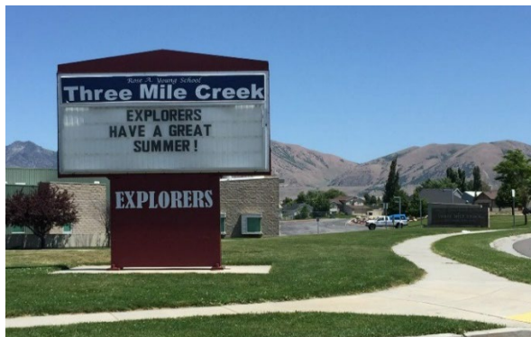
Figure 8: Three Mile Creek Elementary School
