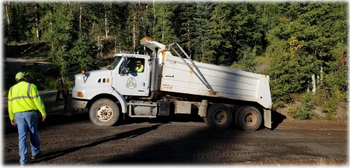
Milling Project Gurr Well Road
