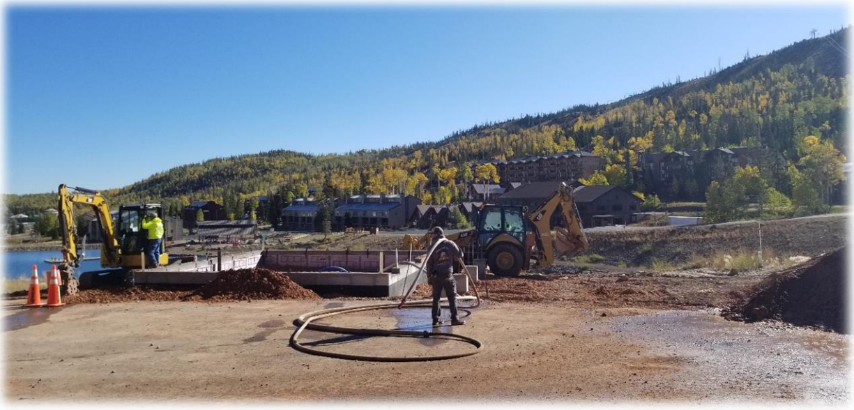
Back Fill Chair One restrooms
