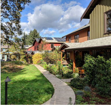
An example of a cottage cluster. A cottage cluster includes smaller homes with a shared open space. Cottage clusters offer reduced landscape maintenance responsibility and efficient parking designs. Cottage clusters provide an opportunity for growth of single-family homes in Midvale.
