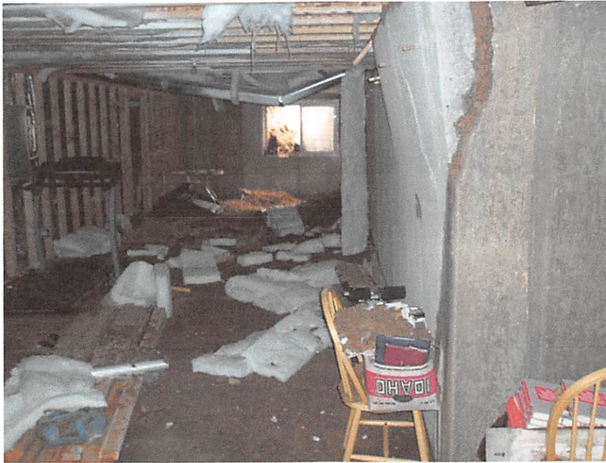
Figure 8. Basement at 1650 East 7687 South showing upper foundation wall (right side of photo) broken by landslide impact.
