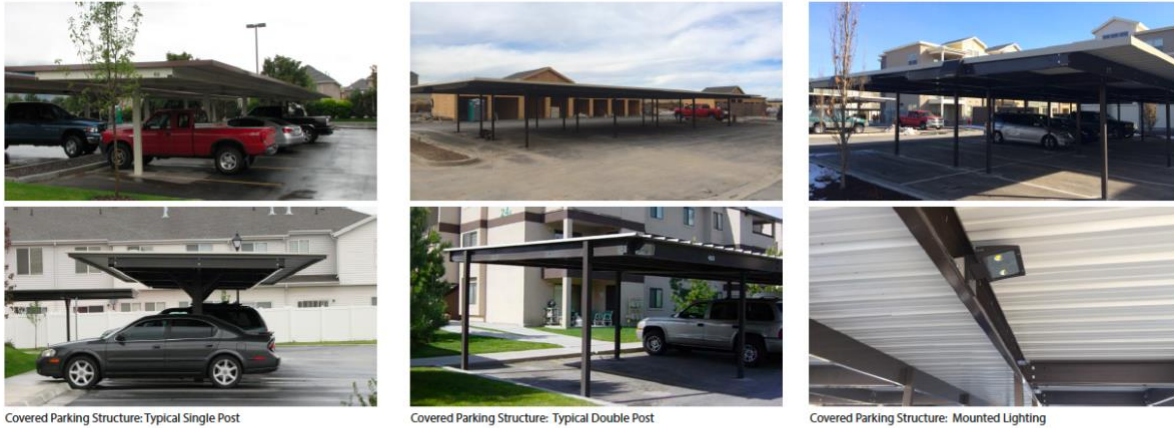
Figure 10: Covered Parking Structures
