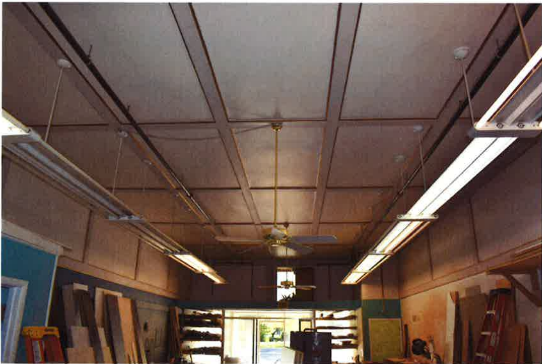
Store Front Ceiling
