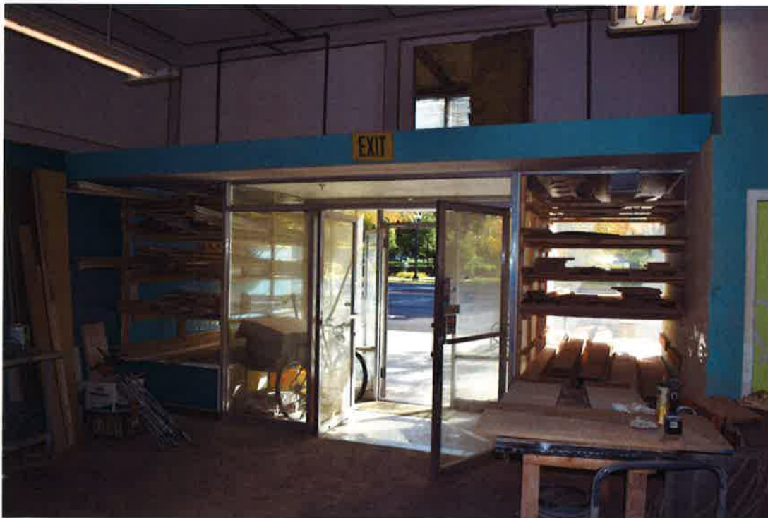
Rear Entrance Interior
