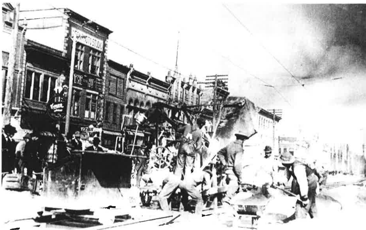
Track Construction along Main Street c. 1911 - The second floors of 41, 45, and 47 N Main can be seen behind the track crew. The Cardon Jewelry pole sign can be seen in front of 41 N Main.
