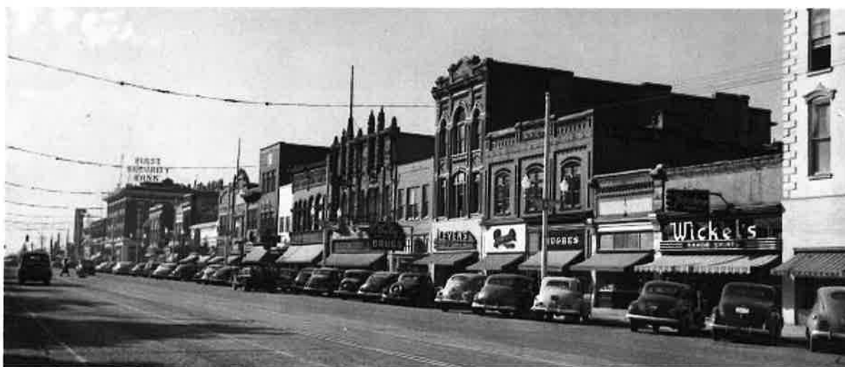
Main Street c. 1940 (Deseret News Photos) - This image of Main Street shows the entire project site from 41 N to 67 N Main.
