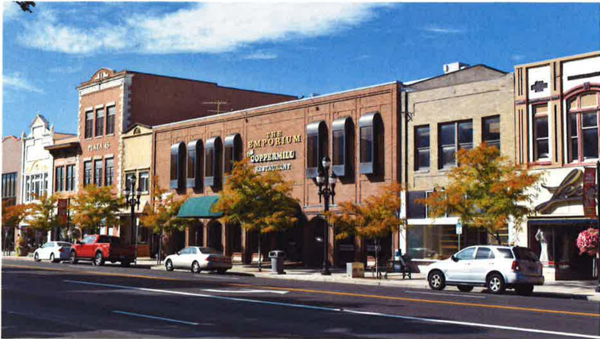
Looking south along Main Street, all the buildings are featured.
