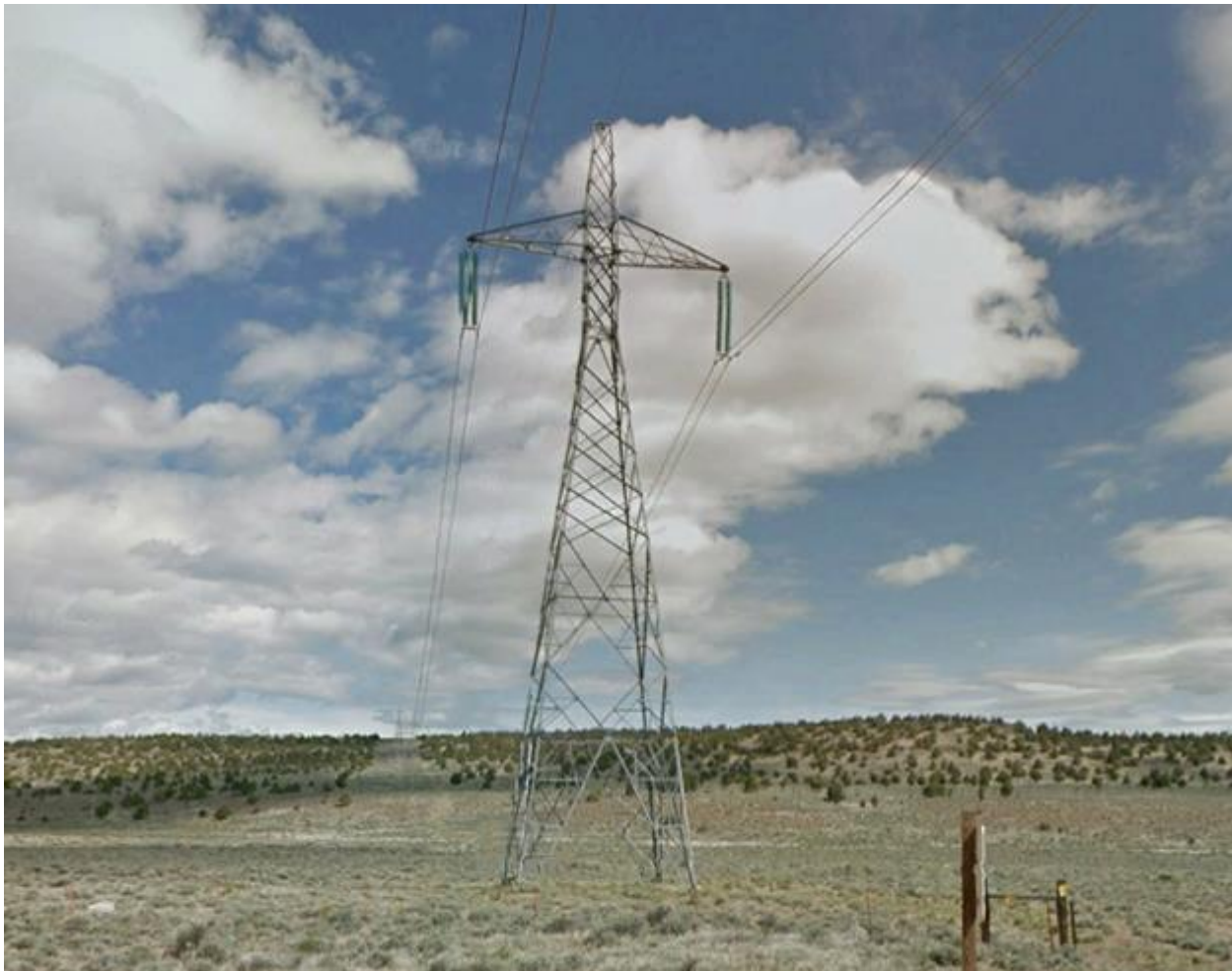
Figure 3. Representative Picture of Self-Supporting I-String Steel Angle or Dead-end Lattice Structure
