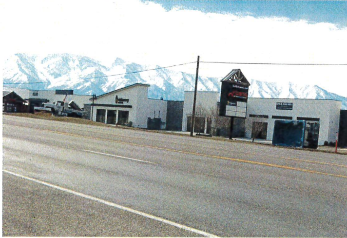
Photos 3-6, Adjacent Properties, Front View
