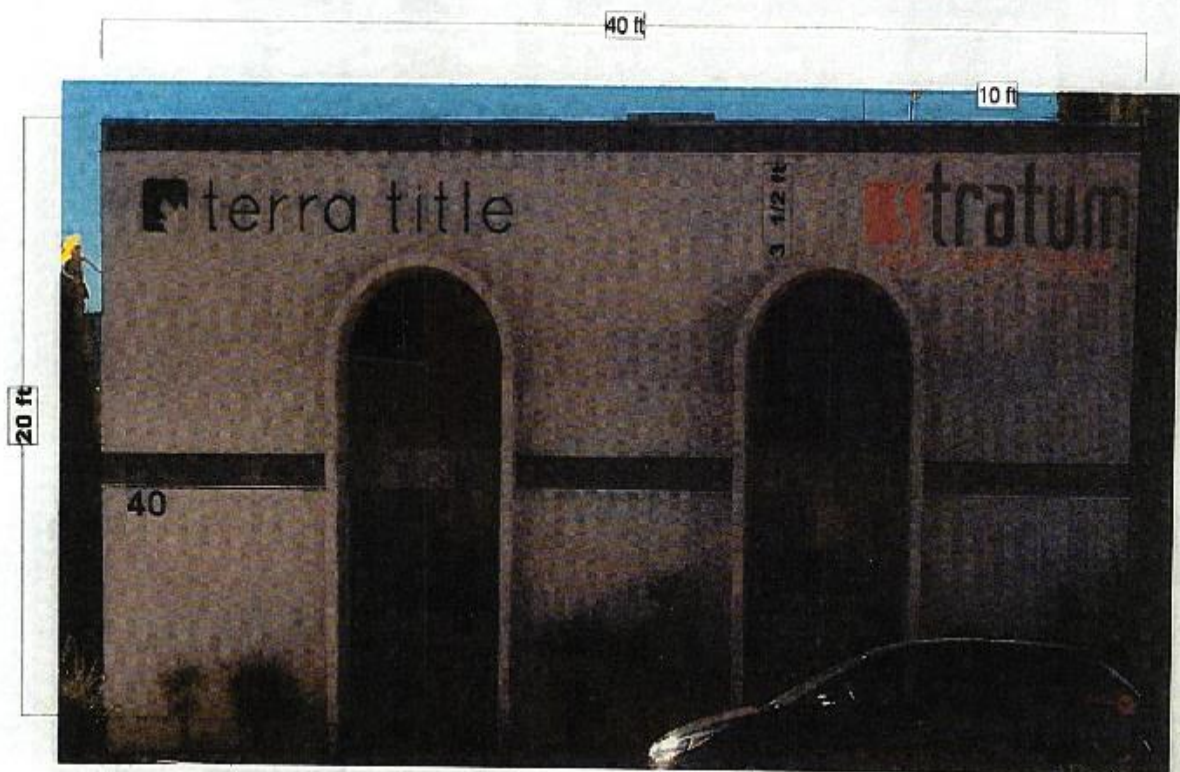
Flat Cut Aluminum Sign with Painted Polyurethane Enamel Finish Stud Mounted to the Wall with 1/2" Stand Offs
