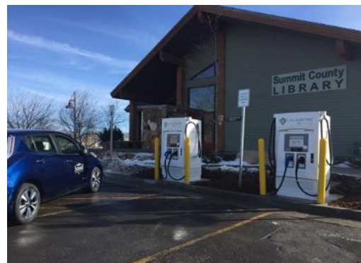
Figure 189. Photo of EV Charging Station at Summit County Library courtesy of Summit County.
