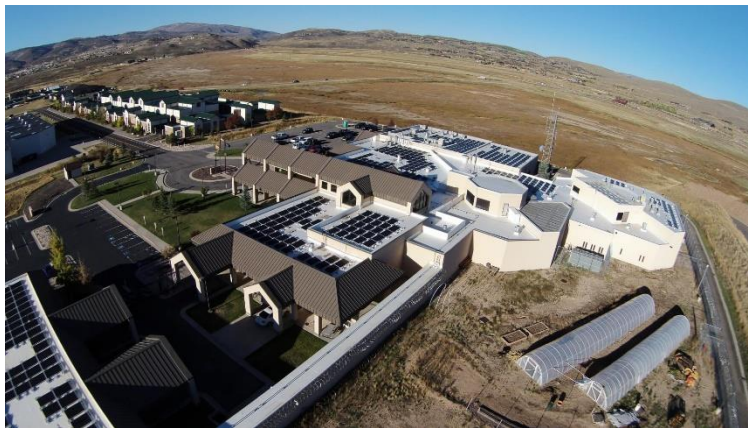
Figure 4. Summit County Justice Center Solar PV Installation (photo provided by Summit County)
