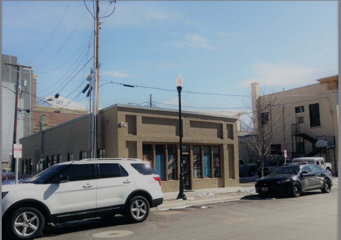
COP Offices located at 48 North 300 West
