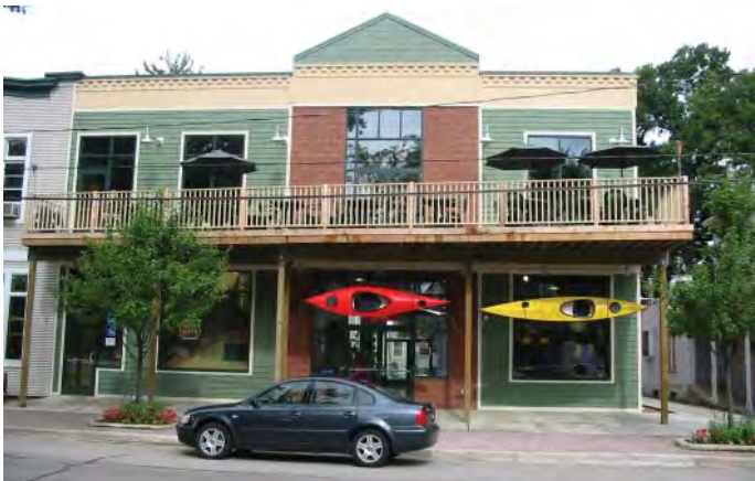
Primary Materials: Painted Wood
