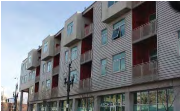
Figure 5.11 (5). Balconies Integral to Facade.
