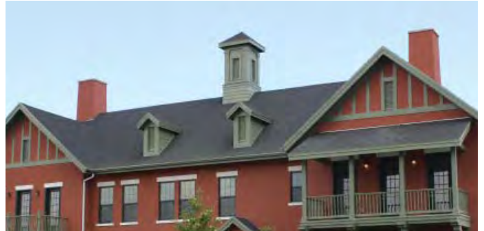
Roof Materials: Asphalt Composite Shingles
