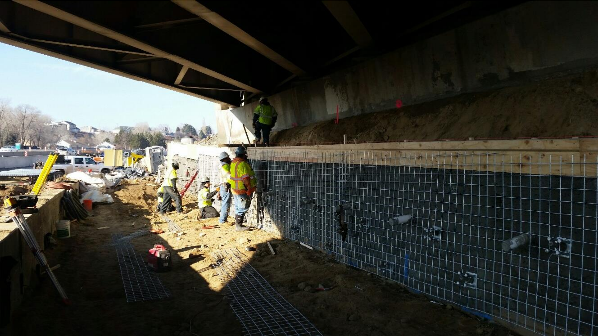
Carterville Road Bridge
