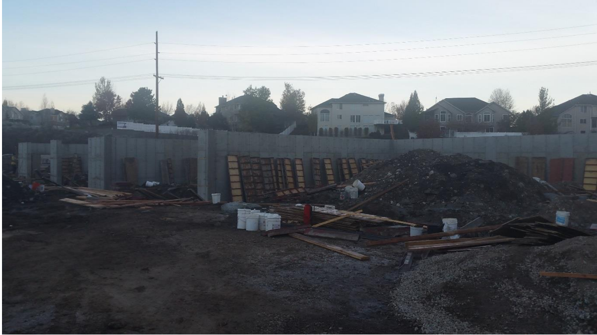
Figure 3- Crews were stripping the forms from the walls over the weekend.
