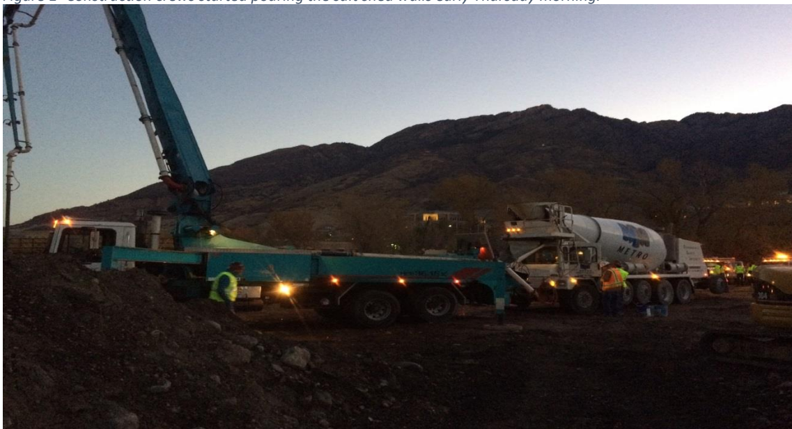
Figure 2- Concrete was pumped into the forms through a pump truck.
