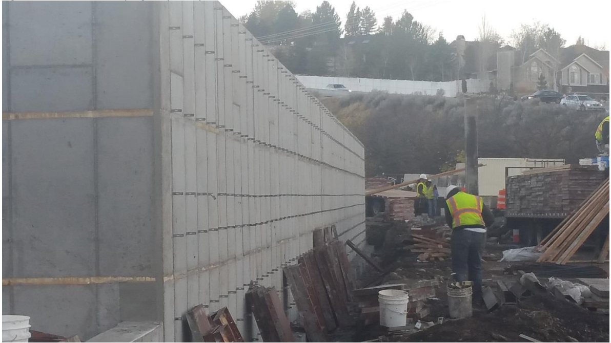
Figure 3- Crews were stripping the forms from the walls over the weekend.
