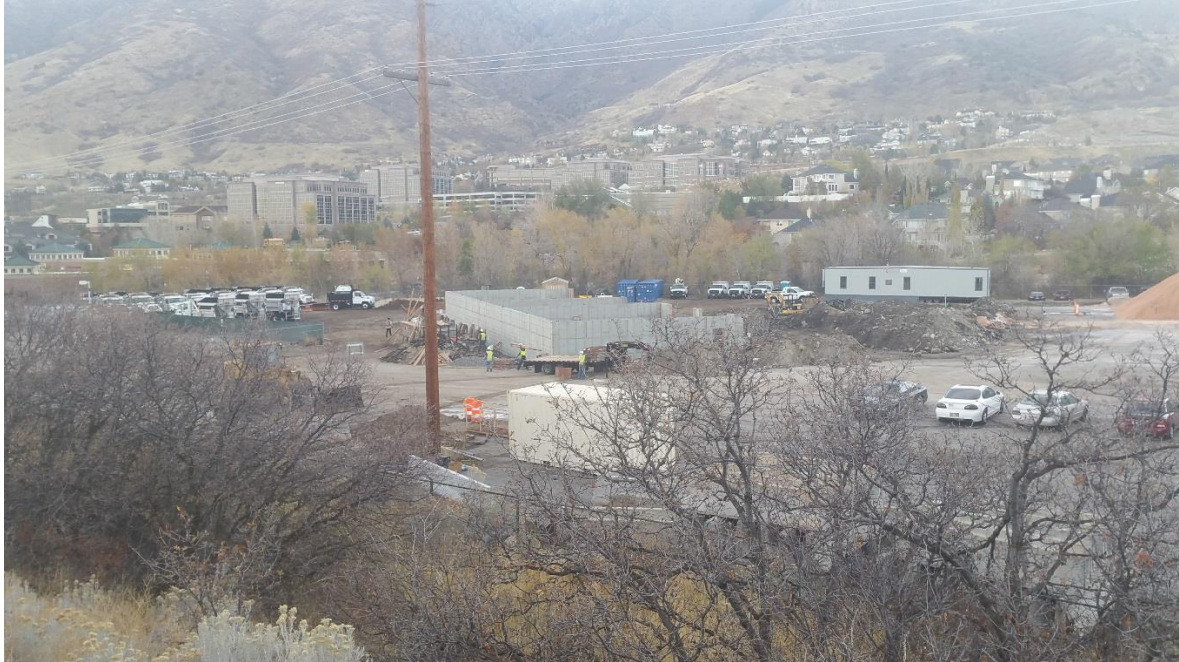
Figure 7- View of the public works site from 3000 East.
