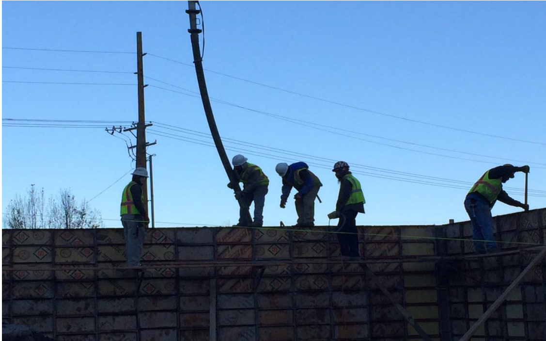
Figure 1- Construction crews started pouring the salt shed walls early Thursday morning.
