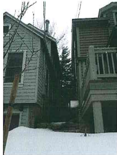
Alley on South side of house
