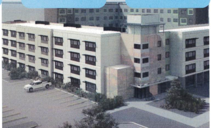
Project Overview: 580 South 500 West, Salt Lake City, UT
