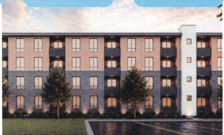
Project Overview: 1776 S West Temple, Salt Lake City, UT
