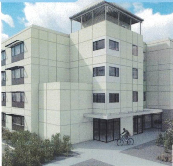
Façade Refresh & Complete Unit Upgrades
