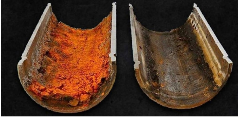
Rust from aging or corroding pipes
