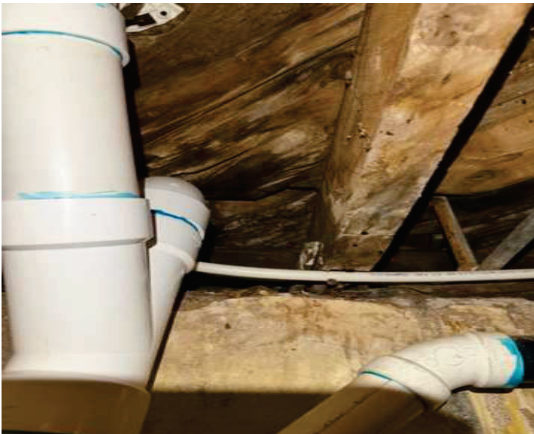
8. Existing Wood Framing in Basement
