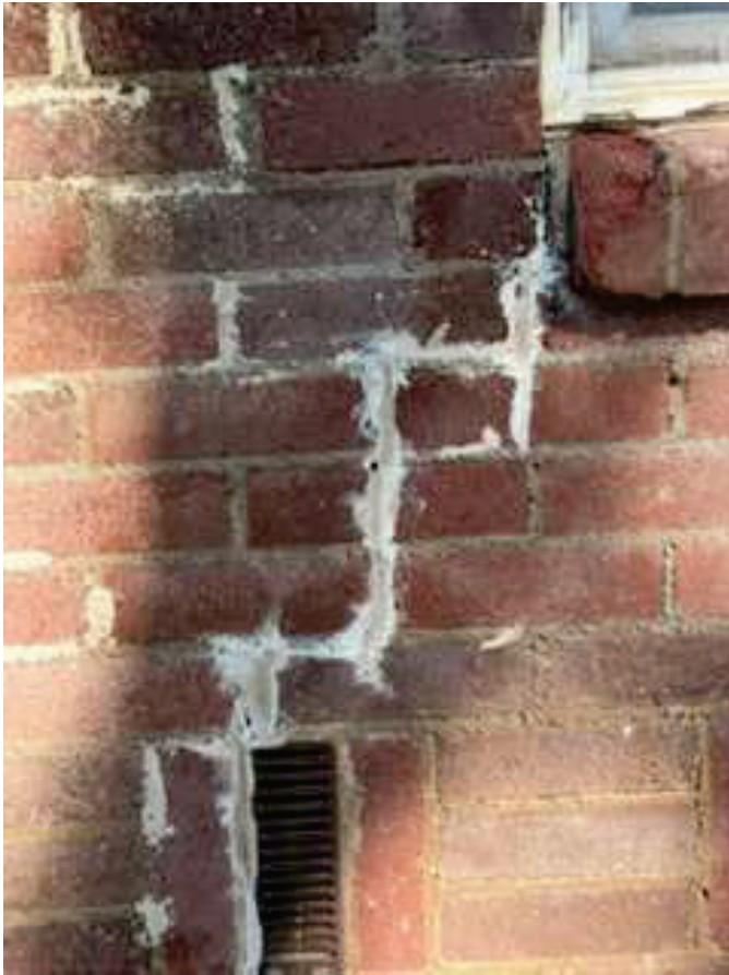
11. Existing Crack Repair in Exterior Brick
