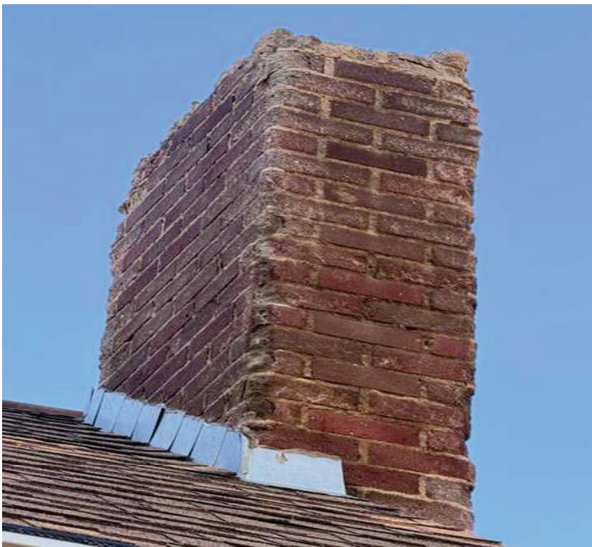
16. Existing Chimney Above Roof
