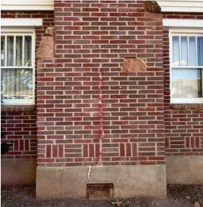
17. Existing Chimney Base
