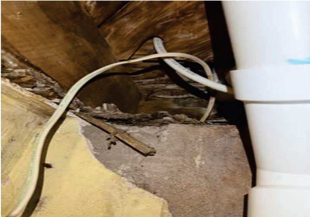
7. Existing Wood Framing in Basement
