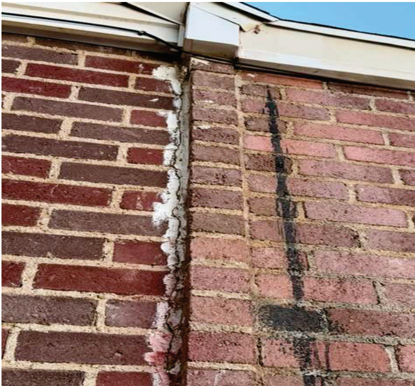
18. Existing Joint Between Original Home & Addition
