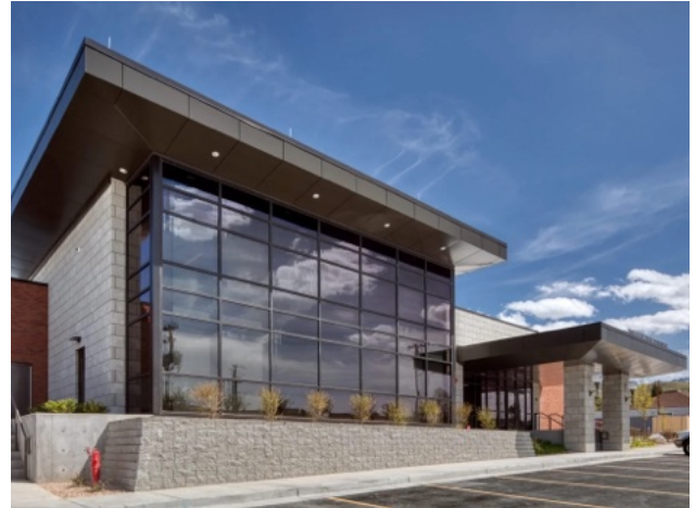
Example Public Facilities: Public Safety Facility Tooele
